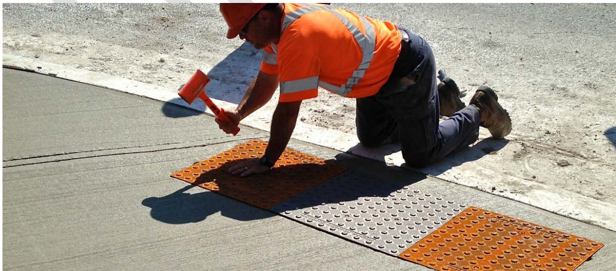
Public Works employee installing a tactile attention indicator in a sidewalk
