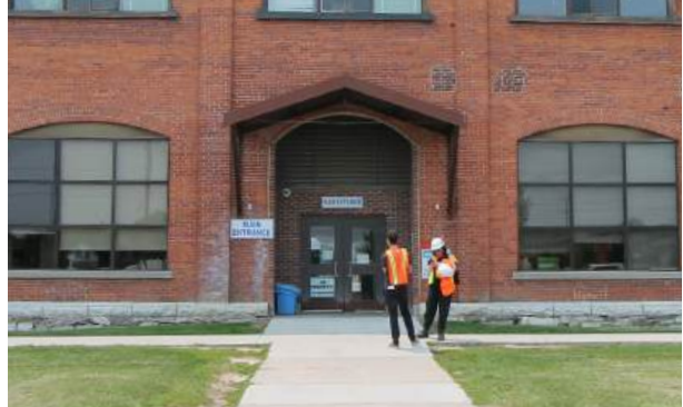
17. Entrance Building 2A (ERA, 2023)
