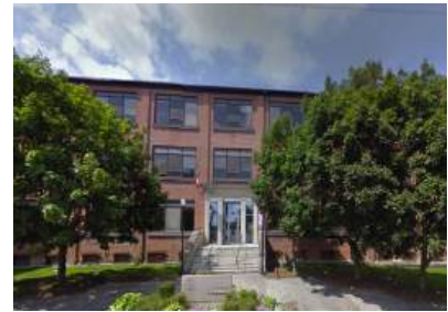
49. Building 2 East Elevation (Google, 2018)
