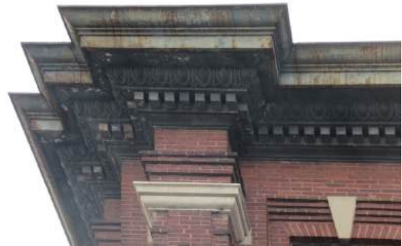
19. Cornice, Building 8A (ERA, 2024)
