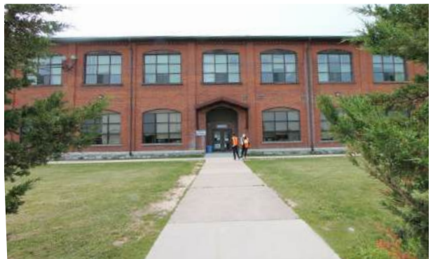
13. Building 2 fenestration (ERA, 2023)
