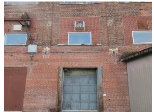
29. Infilled windows and entrances (ERA, 2023)
