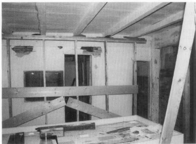
Figure 6. Interior bracing which will last the duration of the mothballing will protect weakened structural members. Jethro Coffin House. Photo: John Milner Architects.
