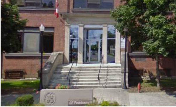
16. Entrance Building 2 (ERA, 2023)
