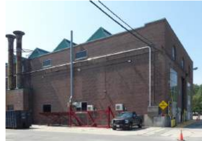
55. West Elevation Building 26 (Source: ERA, 2023)
