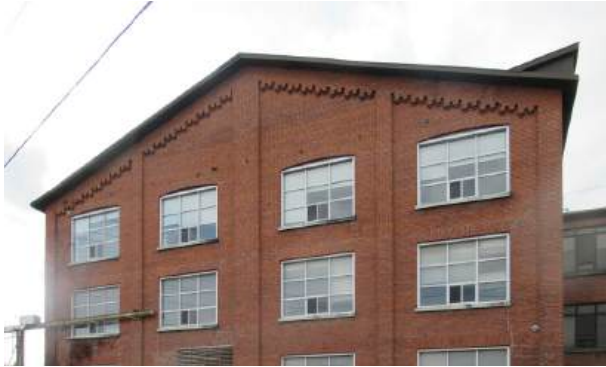
10. Gabled roof and brick corbels Building 30 (ERA, 2024)
