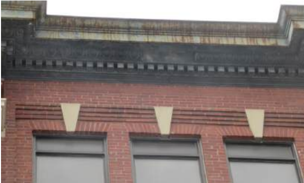
8. Building 8A Decorative brick banding, keystone details (ERA, 2024)
