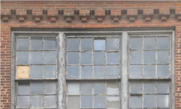
9. Building 30 Decorative brick corbels and original wood windows (ERA, 2024)
