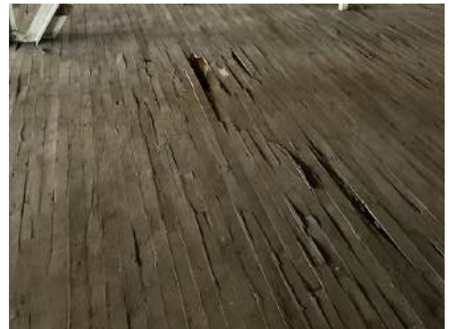
31. Condition of wooden floors (ERA, 2023)
