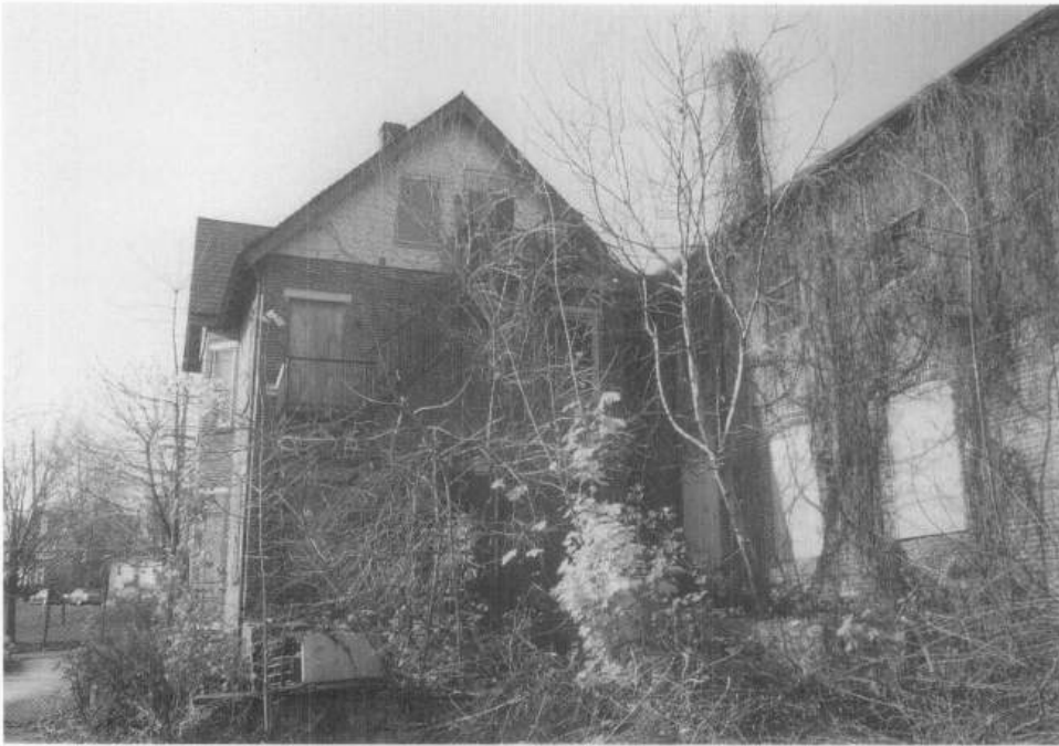
Figure 2. Improper treatment: Boarding up without adequate ventilation, lack of maintenance, and neglect of this property have accelerated deterioration. Photo; NPS file.
