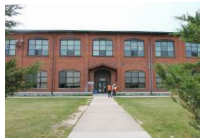
50. Building 2A East Elevation (ERA, 2023)
