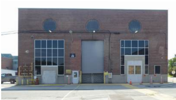
12. Building 26 fenestration (ERA, 2023)
