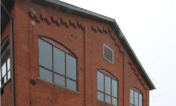
7. Building 30 Victorian Elements (ERA, 2024)
