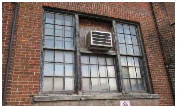
15. Wooden windows on Building 30 (ERA, 2024)
