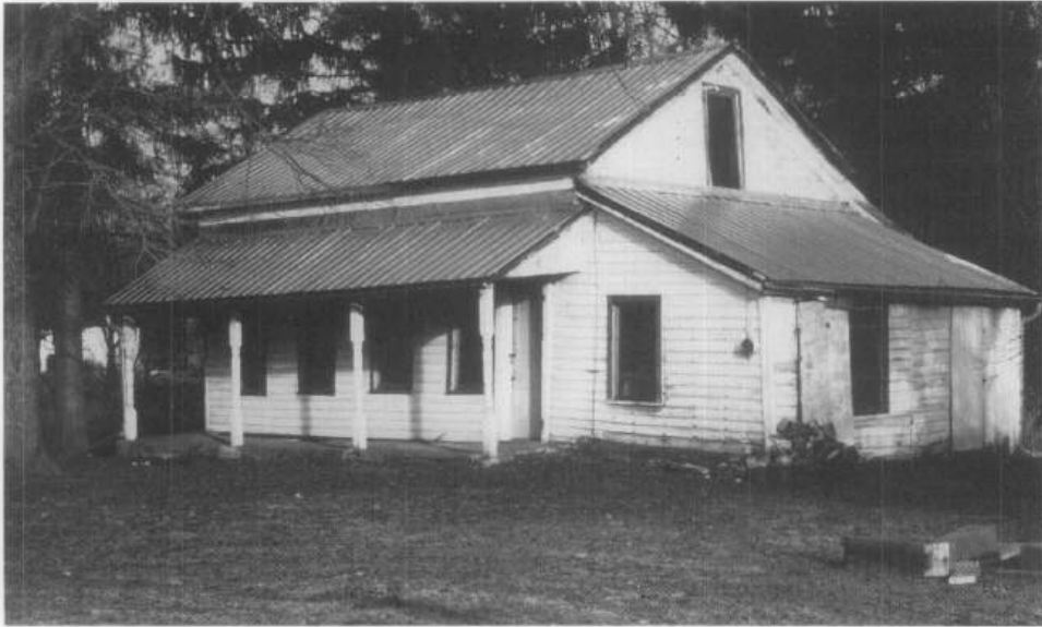
Figure 7. Non-historic materials are appropriate for mothballing projects when they are used to protect historic evidence remaining for future preservation. This lightweight aluminum channel frame and roofing covers the historic wooden shingle roof. Galvanized mesh panels secure the window openings from intrusion by raccoons and other unwanted guests. Photo: Williamsport Preservation Training Center, NPS.
