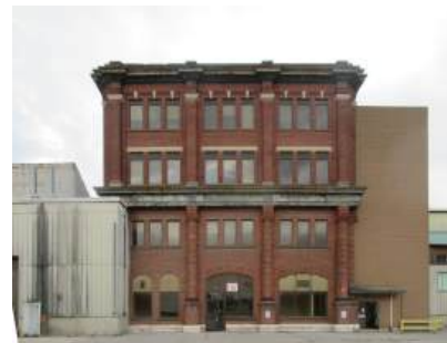
58. East Elevation Building 8A (Source: ERA, 2023)
