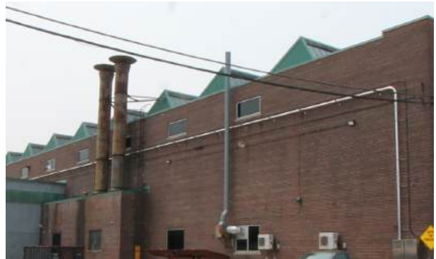
11. Sawtooth roof Building 26 (ERA, 2023)
