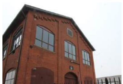
51. Building 2 North Elevation (ERA, 2023)
