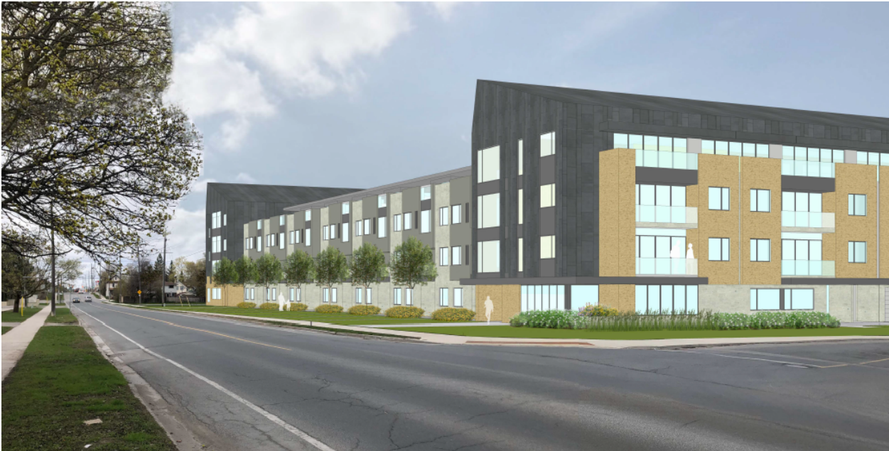
View looking northeast from the intersection of Monaghan Road and Braidwood Avenue.
