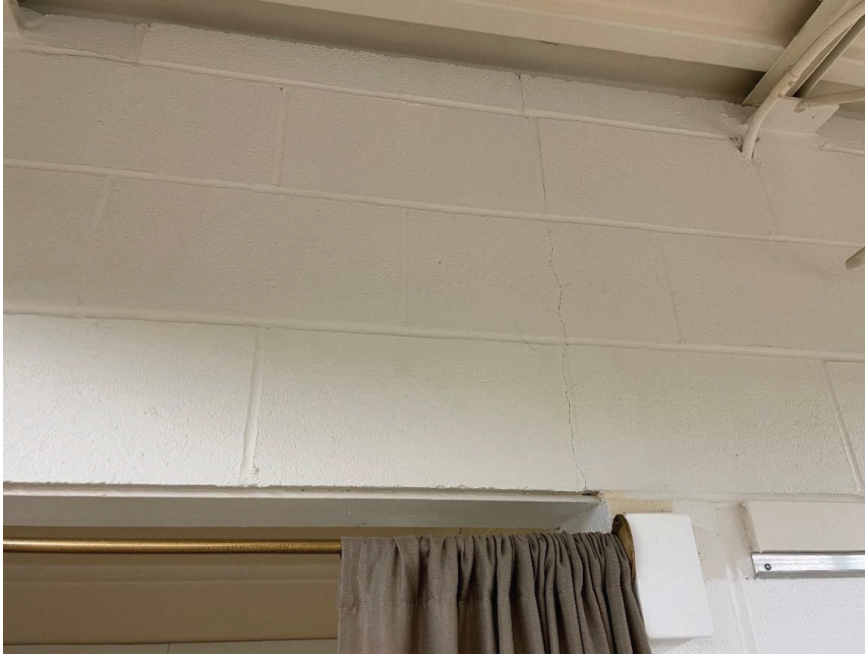
Photo #3 – Vertical crack above corner of interior opening
