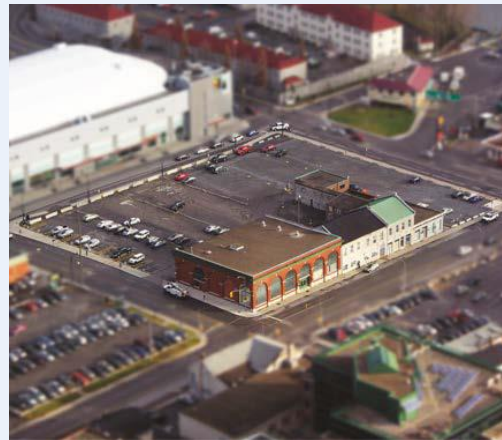
Block 4: Existing Condition
