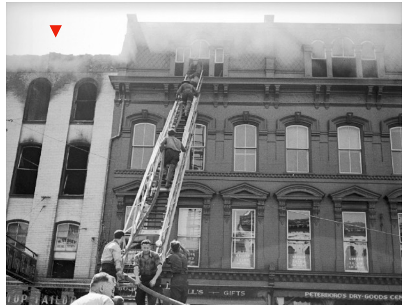
Zack's building (left), showing considerable fire damage and cornice removed. The Cluxton building (right) bearing considerably less damage to the mansard roof above. (Peterborough Museum and Archives.)
