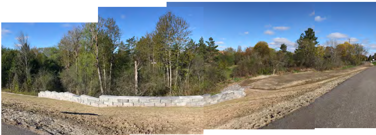
10. A: Views from the adjacent walkway (over the new creek culvert) to the development site, 2019. (BA)
