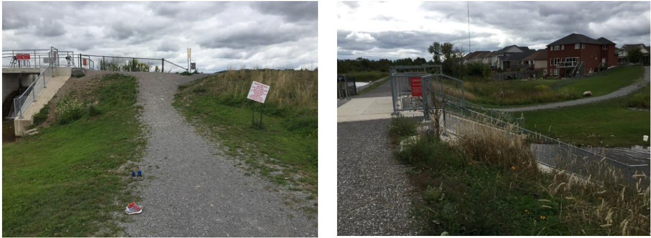
Figure 1 – Existing Walkway Access to Thomson Bay Dam Site
