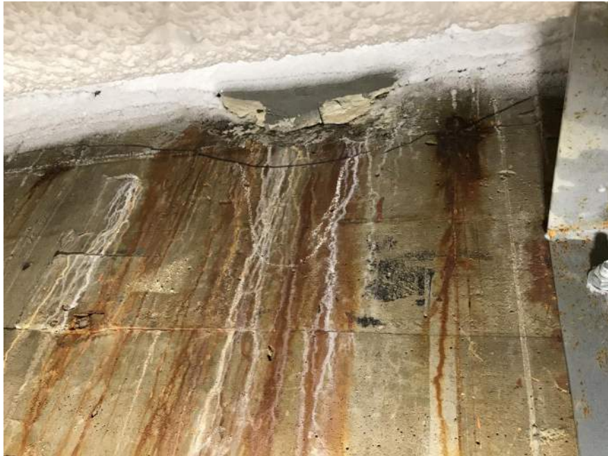
Photograph 9 | Spalled and Delaminated Concrete located towards the Top of the North Foundation Wall in the Brine Trench
