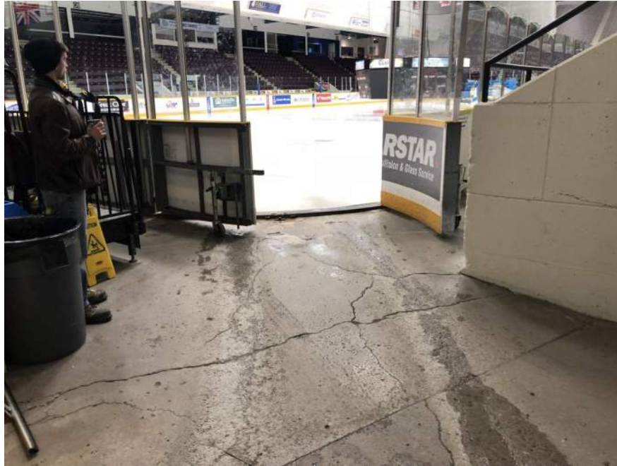
Photograph 1 | Cracking of Existing Concrete Slab along the Ice Resurfacer Path
