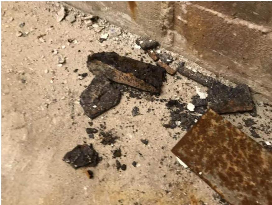
Photograph 14 | Corroded Cast-In Angle Observed on the Crawlspace Floor below the Existing Suspended Slab adjacent to the North Foundation Wall in the Brine Trench
