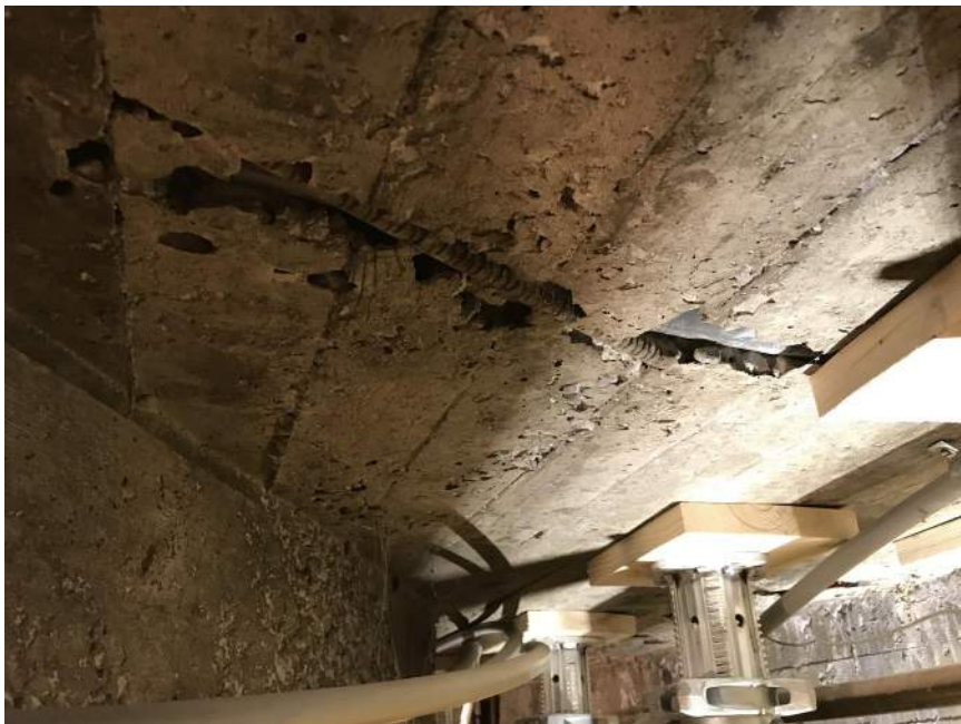
Photograph 6 | Honeycombing and Exposed Conduit Pipe located on the Underside of the Existing Suspended Concrete Slab Beneath the Ice Resurfacer Path
