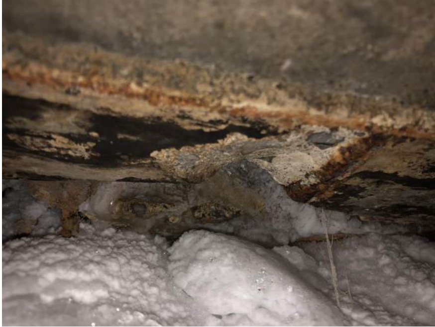
Photograph 13 | Corroded Cast-In Angle on the Underside of the Existing Suspended Slab adjacent to the North Foundation Wall in the Brine Trench
