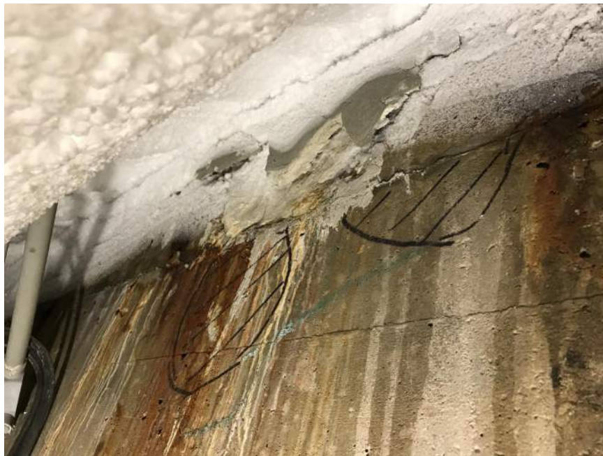
Photograph 8 | Spalled and Delaminated Concrete located towards the Top of the North Foundation Wall in the Brine Trench
