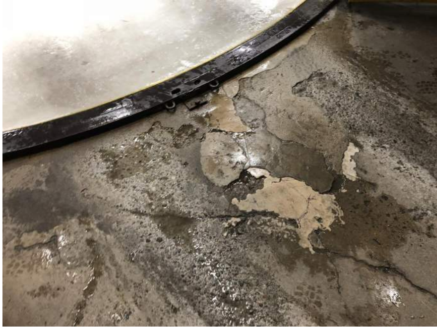
Photograph 3 | Cracking and Delaminating Concrete adjacent to the Dasher Boards along the Ice Resurfacer Path (Southeast Corner of the Ice Rink)
