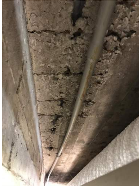
Photograph 11 | Honeycombed Concrete and Exposed Reinforcing Bars along the Underside of the Existing Concrete Slab Adjacent to the South Foundation Wall in the Brine Trench
