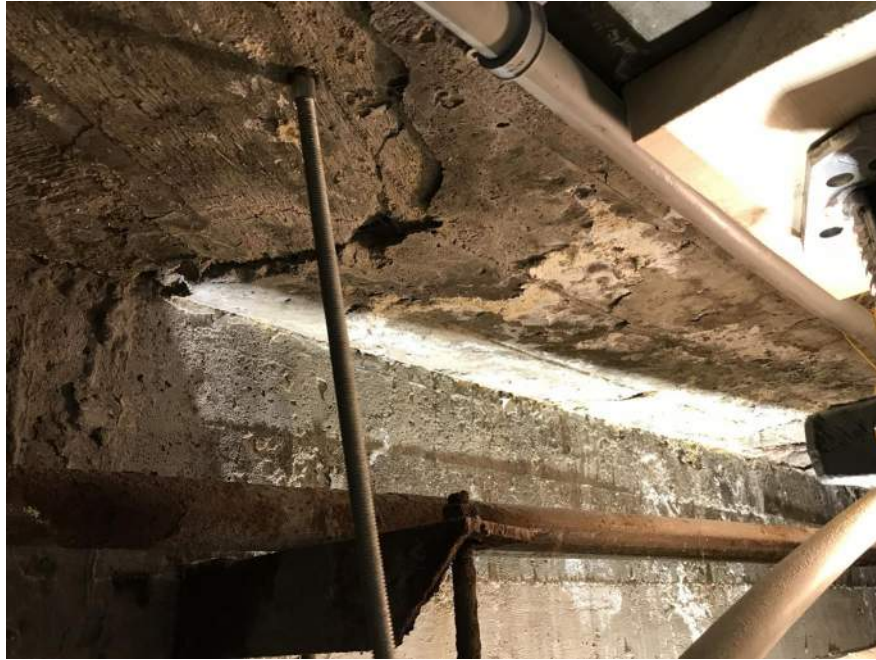
Photograph 7 | Cracking located on the Underside of the Existing Suspended Concrete Slab Beneath the Ice Resurfacer Path
