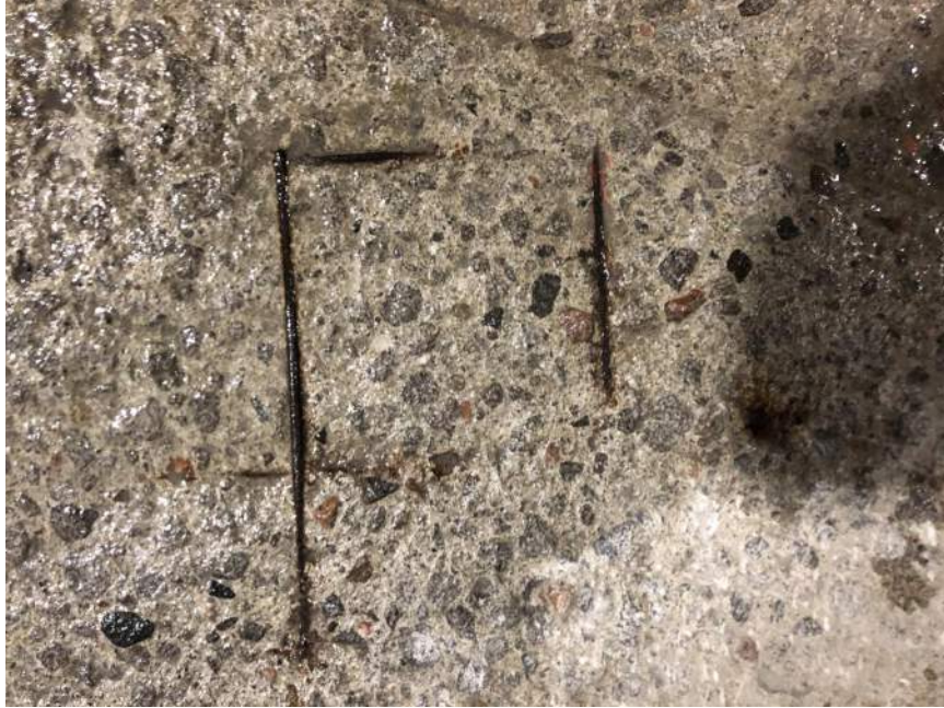
Photograph 5 | Exposed and Corroding Wire Mesh in the Topping Slab located along the Ice Resurfacer Path
