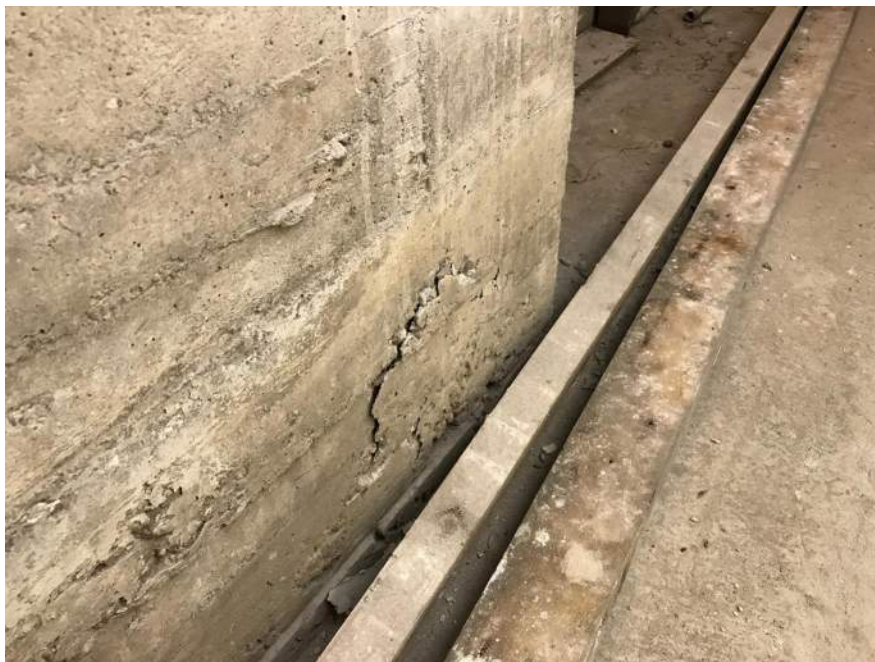
Photograph 10 | Spalled and Delaminated Concrete located at the bottom of the South Foundation Wall in the Brine Trench
