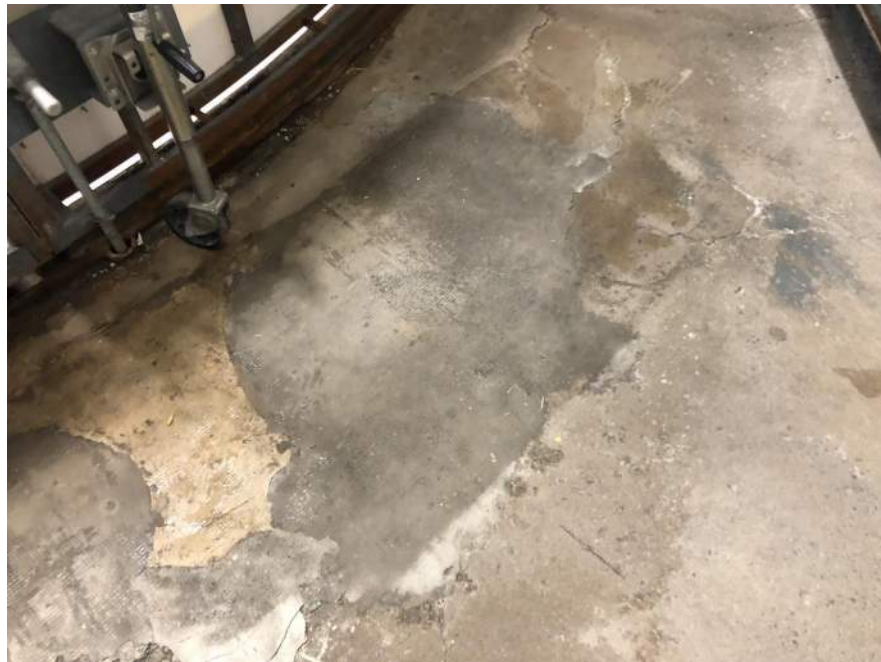
Photograph 4 | Cracking and Delaminating Concrete adjacent to the Dasher Boards at the Alternate Ice Resurfacer Doors (Southwest Corner of the Ice Rink)
