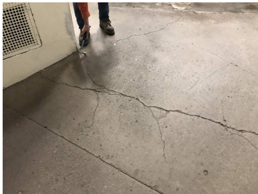
Photograph 2 | Cracking of Existing Concrete Slab along the Southwest Corner of the Ice Rink
