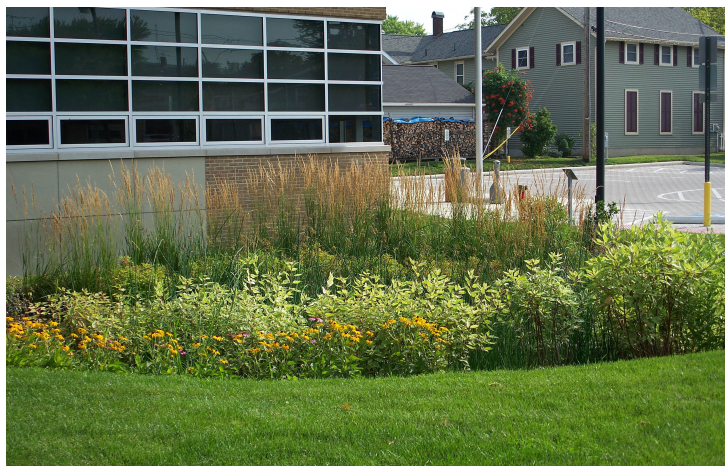
Rain garden capturing runoff from building roof
