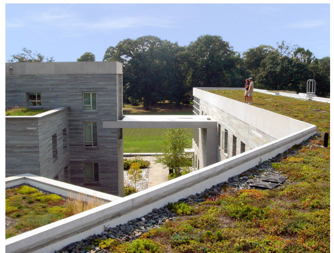
Green roofs help to reduce energy consumption by providing natural cooling in the summer months.
