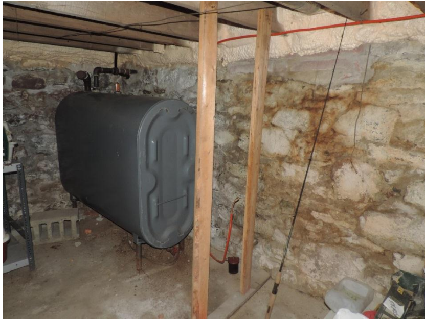
Plate 40: Wood beams and stone foundation in basement of main residence
