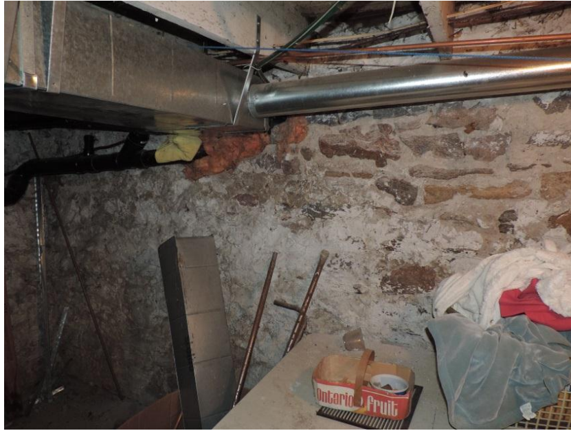
Plate 19 North basement wall showing stone foundation
