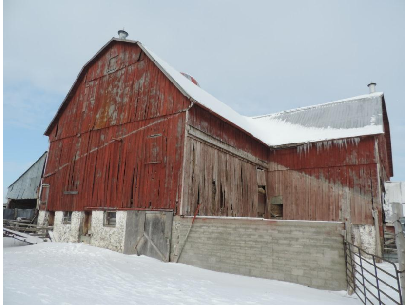
Plate 21: Southeast view of timber bank barn showing steel roof and cupolas
