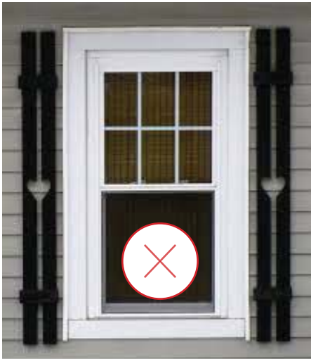
63. Incorrectly proportioned new shutters. (Source: oldhouseguy.com)
