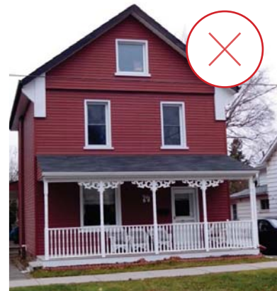
41. Synthetic vinyl siding conceals original cladding and architectural detailing and is also not appropriate for the architectural style of this building. (Source: ERA)
