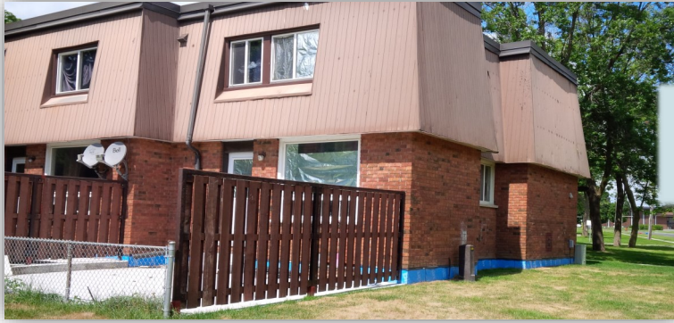
Major foundation repair at 999 Hilliard Street
