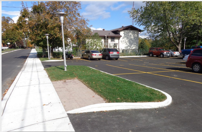
Parking Lot Expansion and drainage 53 Spring Street, Norwood
