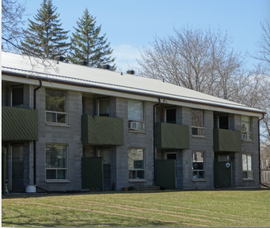
Roof Replacement 8 Victoria Street, Havelock
