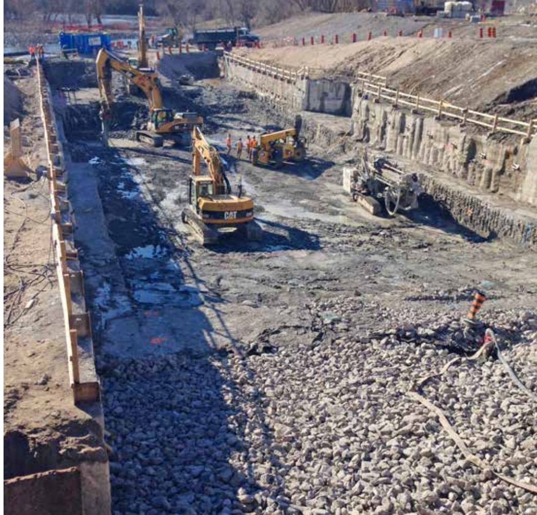
Excavation work to upgrade the London Street Generating Station.
